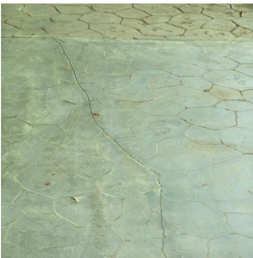
Crack in Pavilion Floor
